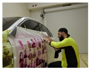
Vehicle graphics should not be applied to a newly painted vehicle. Allow at least 60 days for fresh paint to cure.
